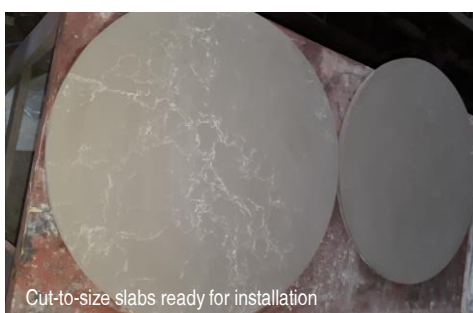
Slabs cut-to-size on CNC Machine (off-site)
