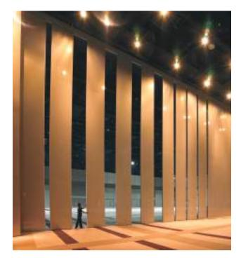
Hotels and Malls can use movable walls to create more number of functional areas within the available space – for instance, a banquet hall or a convention centre in a Hotel can double up with a movable wall partition to accommodate two functions or conferences simultaneously.
